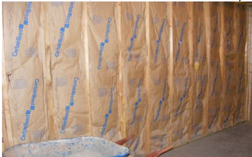
Example of interior framing in the basement with craft paper
